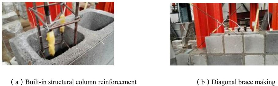
( a ) Built-in structural column reinforcement
